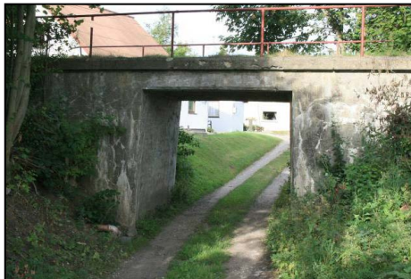
Bro for Ågårdsvej over banen, km. 20,0
